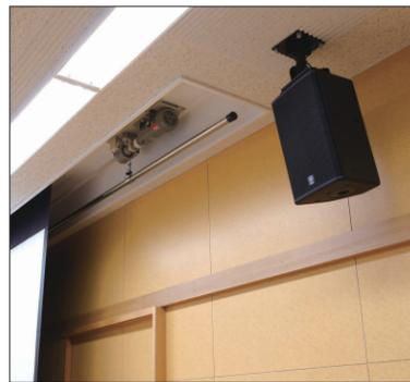
For maximum flexibility the three basically independent sound systems provided in the large lecture hall and two smaller lecture rooms are linked via a Cobranet network that allows audio from the large hall to be monitored in either or both of the smaller rooms, while questions from the smaller rooms can be monitored and answered by the lecturer in the large hall.
