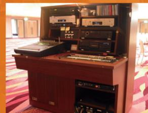
Similar systems, including the O1V96 console, are provided in the control room and in a movable rack located in the hall itself. Wall-mounted connectors, including connectors for the Cobranet Ethernet cables, minimize the need for long cable runs around the room. The DME24N is mounted in a rack in the control room along with four AD8HR AD converters, an NHB32-C digital audio interface, and six P2500S power amplifiers.
